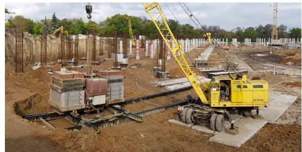
Figure 5. Coordinate piling method by using two modules with their sequential reconnection
